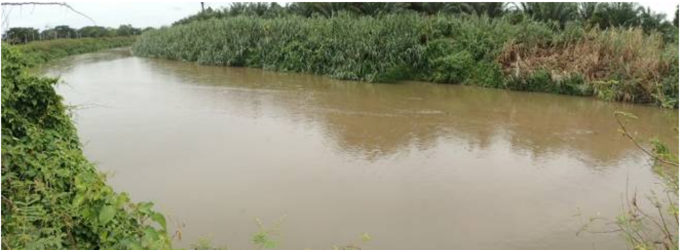
Figure 12. Zone C is located in 4° 20' 3.6378", 101° 5' 20.3352" and the environment may be typically characterised by riparian clearings and channel straightening. Steep banks and failures were prominent. Sediment deposition, sandy and muddy substrates have caused the channel to be shallow in certain parts. The mean average water physico-chemistry values (n=36, mean±SD) measured were DO = 6.80±0.59 mg/L; BOD 5 = 7.25±3.02 mg/L; COD = 21.17±0.19 mg/L; pH = 7.06±0.32; TSS = 43.22±29.14 mg/L; TUR 57.42±37.65 FAU; AN = 0.0608±0.0483 mg/L; FE = 0.5944±0.3666 mg/L; NO 2 -N = 0.0164±0.0097 mg/L; NO 3 -N = 5.12±2.38 mg/L; PO 4 = 0.2294±0.0961 mg/L; and SO 4 = 2.19±1.78 mg/L.
