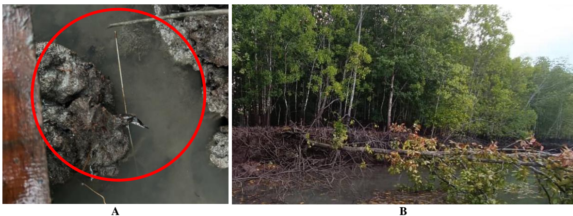
Figure 7. A sediment cluster was found near the bank's bottom with: A. An erosion pin detached with it, indicating the bank failure; and B. Mangrove tree uprooting due to the bank failure at station T1
